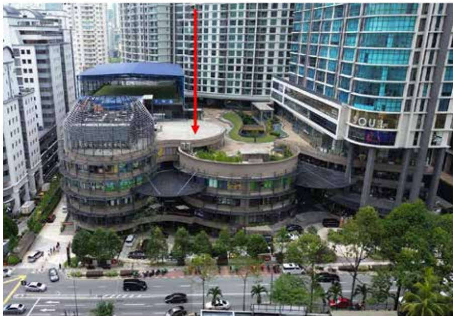
AN AERIAL VIEW OF THE SUBJECT PROPERTY – A STRATIFIED SEVEN (7) STOREY SHOPPING CENTRE KNOWN AS 163 RETAIL PARK
